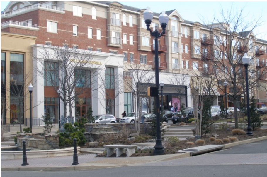
Mixed-Use Transit-Oriented Development in Arlington County, Virginia Photo credit: Jana Lynott
